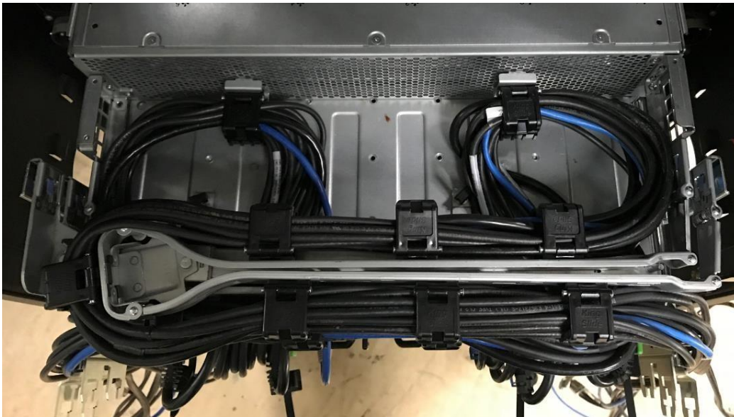
Figure 61: Open Status of Routing the Cables 2
