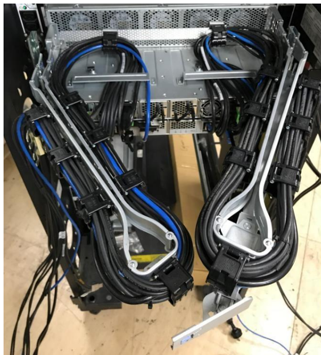
Figure 60: Open Status of Routing the cables
